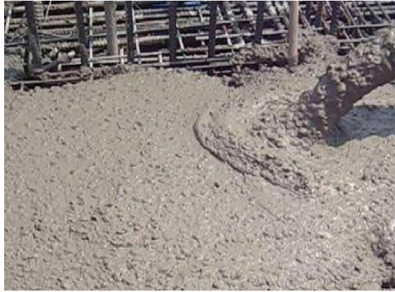
Self Compacting Concrete
