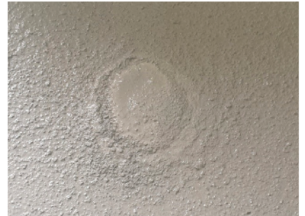
Flowable Fill Foam Concrete
